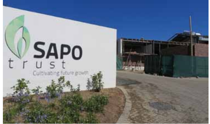
Alterations at the outside of the existing store.
